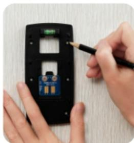
*Note: Use the provided screws with anchors when mounting on brick, concrete, or stucco. When mounting on wood or vinyl, you may use the screws directly without anchors.*
